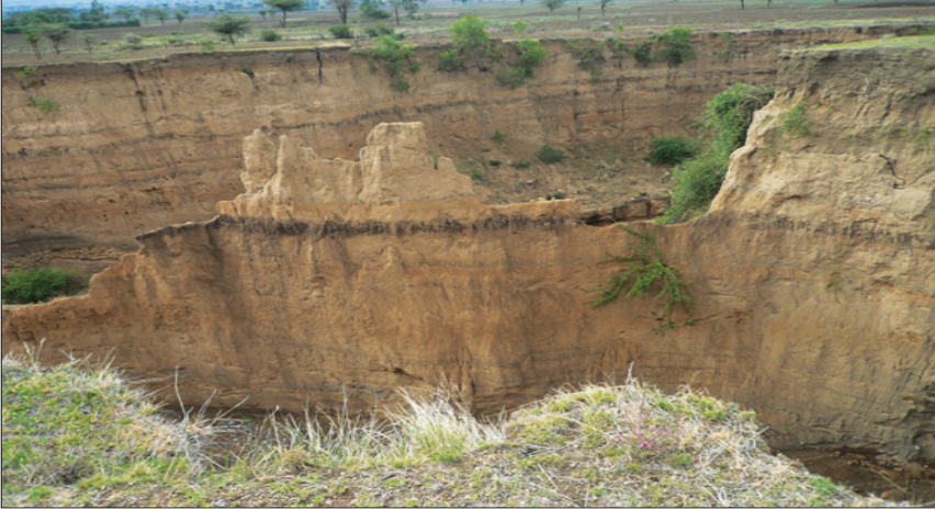
Figure 2.15: Gully erosion This very deep gully developed because of the construction of the main road at Kurfa, past Nazareth (Adama), on the way to the town of Wolenchiti, Oromia Region.
